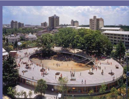
An example of green building found at a Nursery School in Tokyo.
