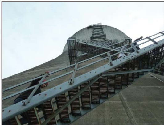
Looking up the cooling tower
