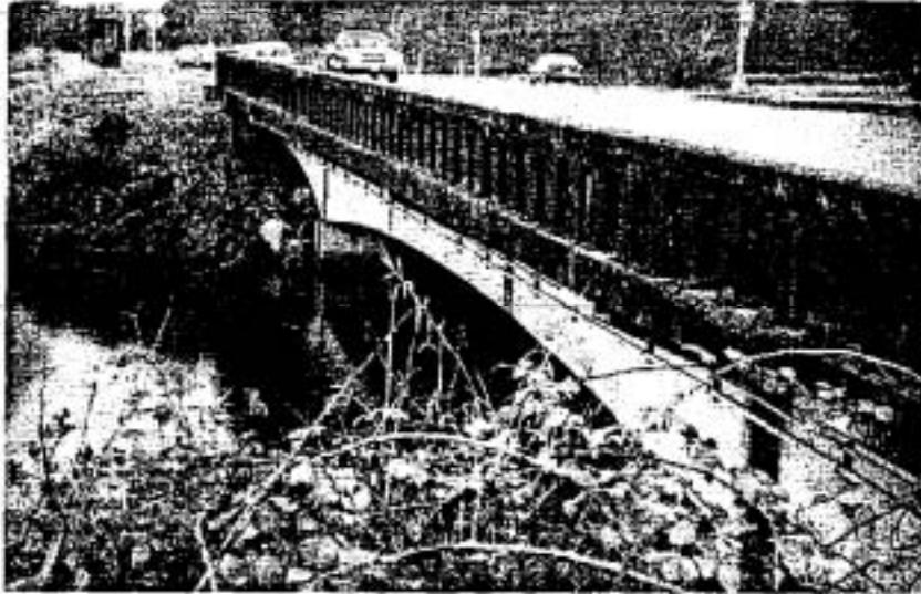
Photograph 5: Percival Bridge - Looking Upstream
