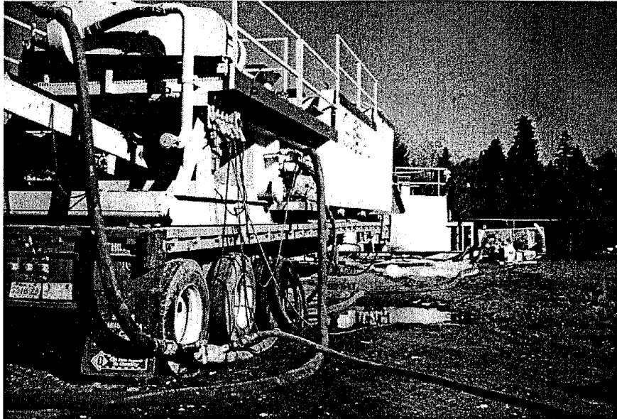
Figure 6 Mechanical Dewatering - Centrifuge and Associated Equipment for Hydraulically Dredged Material
