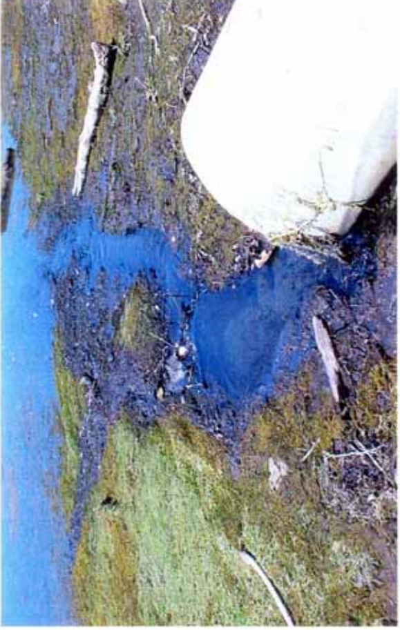
7th Avenue outfall 7/23/02
