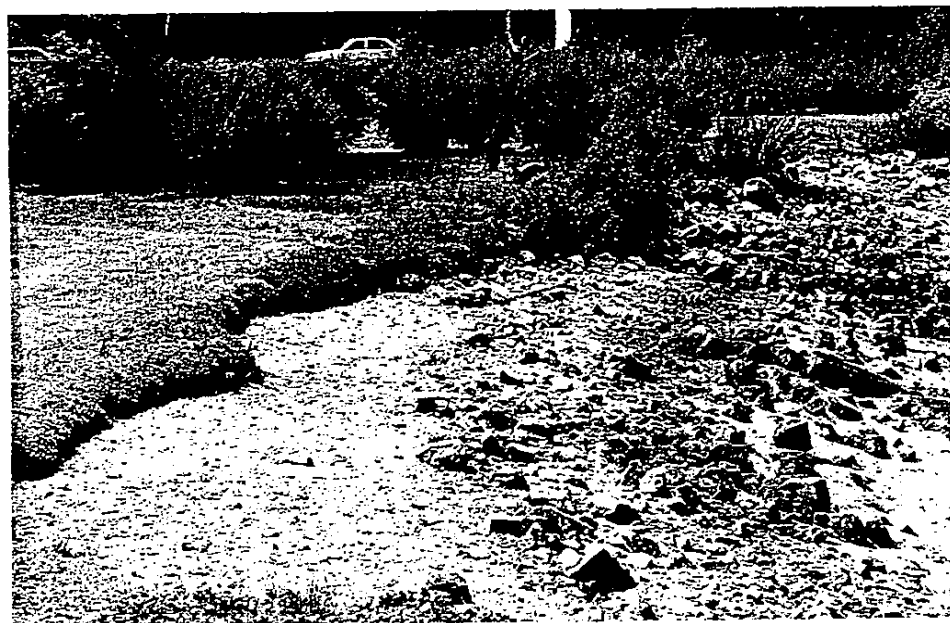
Photo 3 Zone 1 Beach erosion at Marathon Park
