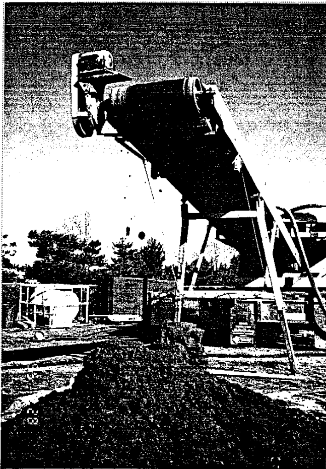
Figure 11 Conveyor and Sediment Storage
