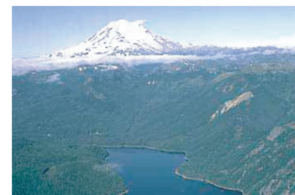
Bumping Lake Dam
