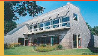
Giltsland Farm, Maine. (Hydronically heated)
