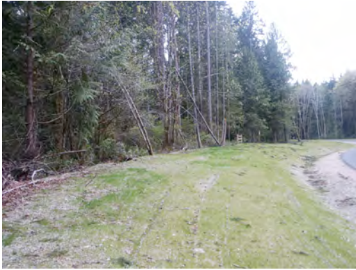
Plate 8: Road Construction Adjacent to Wetland Buffer at Cooper Point
