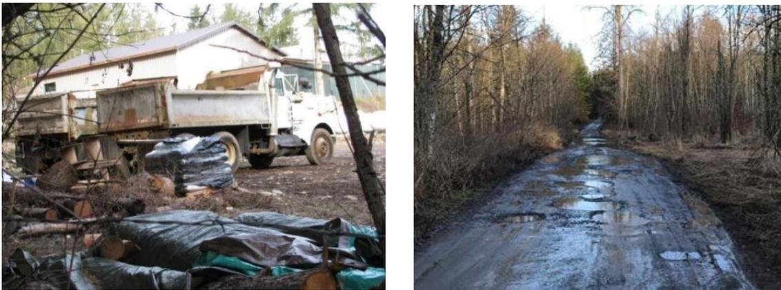
Figure 15: Degraded easement from increased traffic. Truck, heavy equipment, and marijuana worker traffic significantly degraded road conditions on this single-lane easement outside Yelm, Washington. (Photographs by author, 2017).
