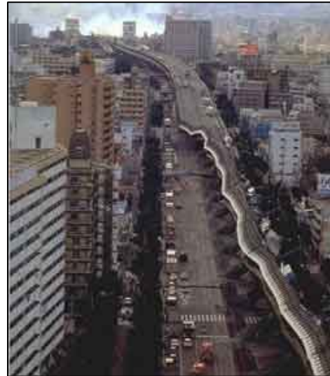
Figure 7: Roads in Kobe, Japan
