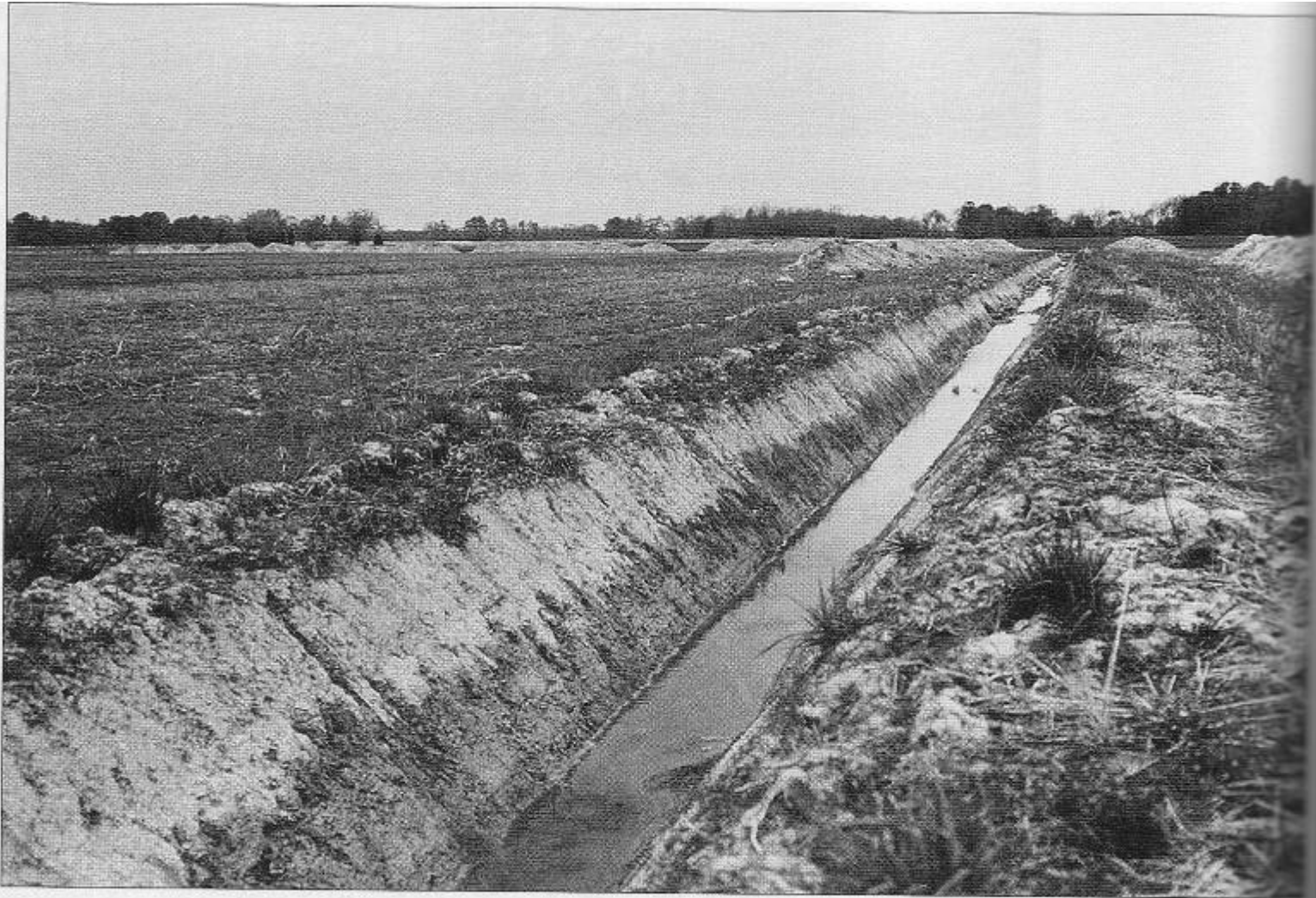
FIGURE 6.35 An open-ditch drainage system designed to lower the water table during the wet season. The water flowing in the ditch has seeped in from the saturated soil. Such ditches also speed the
