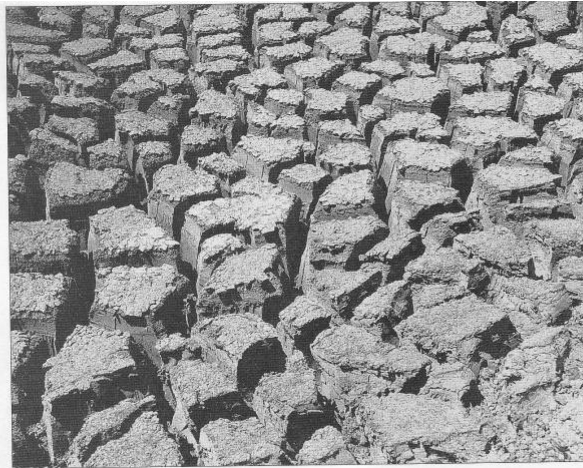
FIGURE 4.43 Certain types of clays, especially the smectites, undergo significant volume changes in conjunction with changes in water content. Here, an expansive soil rich in smectite clay has shrunk during a dry period, causing a network of large cracks to open up in the soil surface. (Courtesy of USDA Natural Resources Conservation Service)
